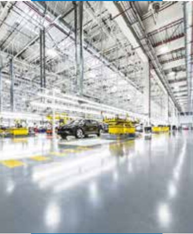
Fiber reinforced Concrete floor with Mapecofibre ST 42
