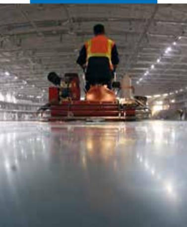
Fiber reinforced Concrete floor with Mapecofibre ST 42
